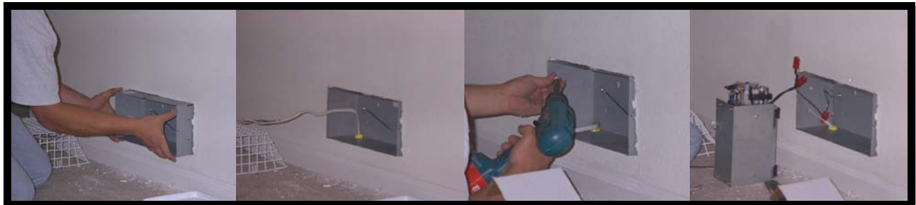
Insert can into wall.
