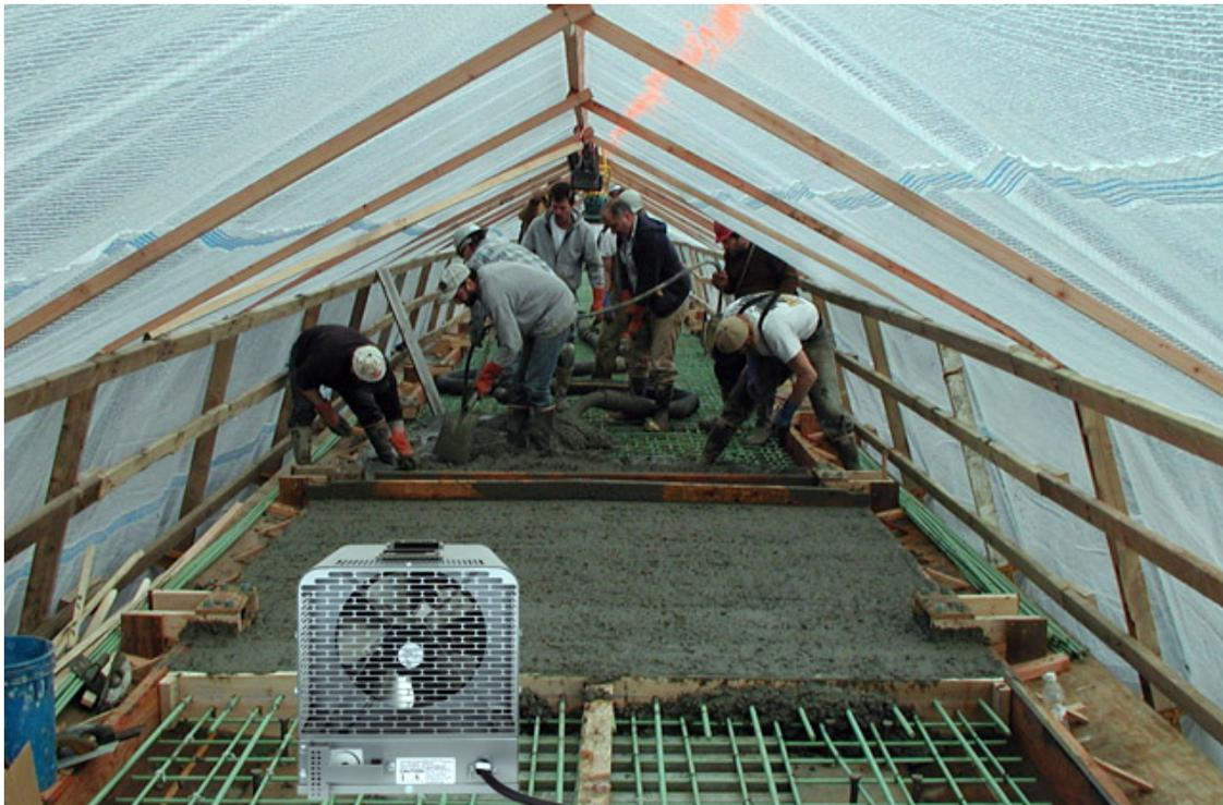
Curing is an essential part of using concrete during construction. Done correctly it will increase the concrete's strength and durability.
