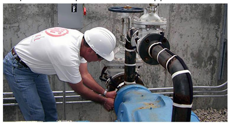
In cold climates, insulation alone often fails to prevent pipes from freezing. A well-designed and installed pipe freeze protection system ensures continuous water flow and prevents costly building damage.
