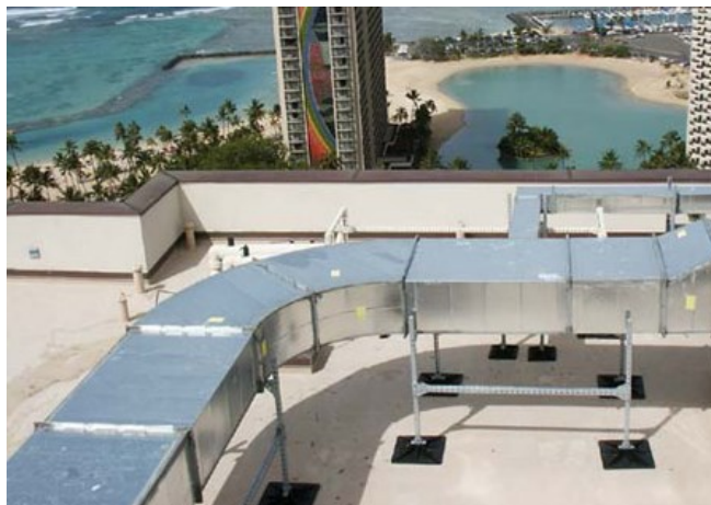
Ducted Roof Top
