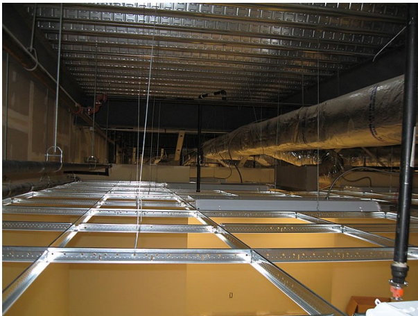
Drop Ceiling Plenum
