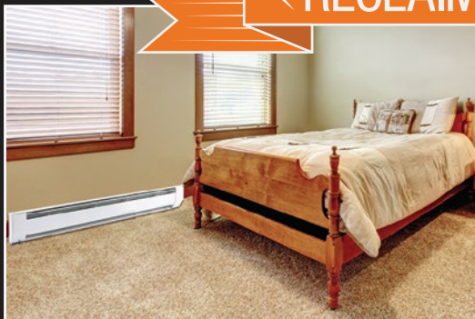
Standard Baseboard Heater
